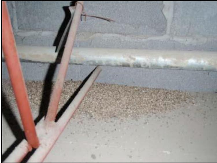
Vermiculite insulation has leaked from the masonry walls.
